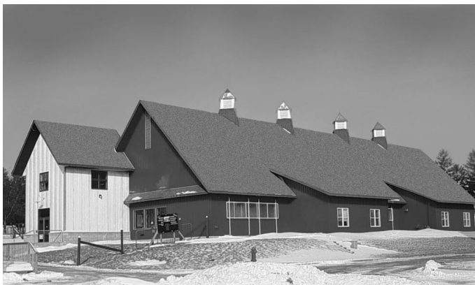
Construction of a new Cattle and Horse Barn was completed in December.
